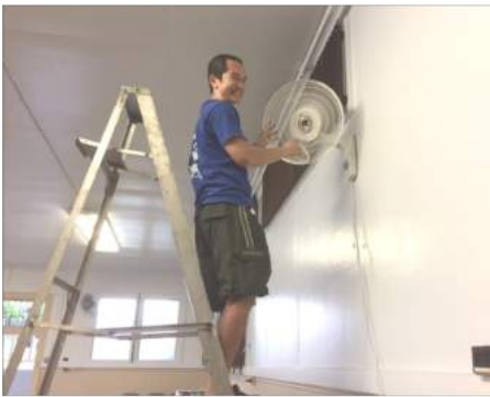
Isaiah Nakano removes fan for cleaning
